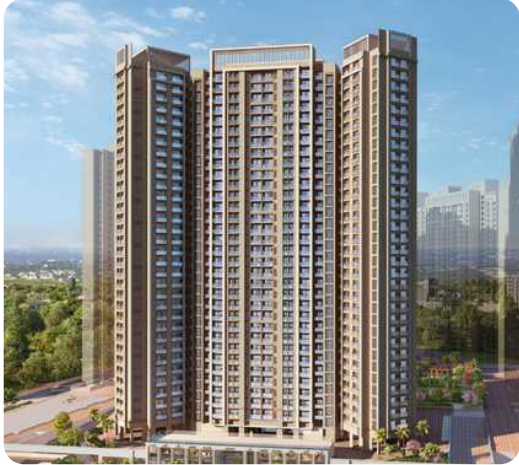
Dosti West County Project, Thane 8 Towers, 30 Floors | Residential Project Firefighting Work
