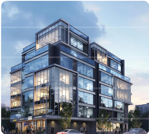
Mahant Chamber, Thane 6 floors | Commercial Project Electrical & Firefighting Work
