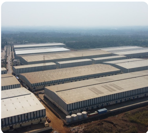
Antariksha Logipark, Dohale, Bhiwandi Warehouse Firefighting Work
