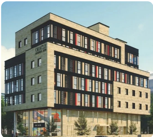
Oracle Business Hub, Thane 6 floors | Commercial Project Electrical Work
