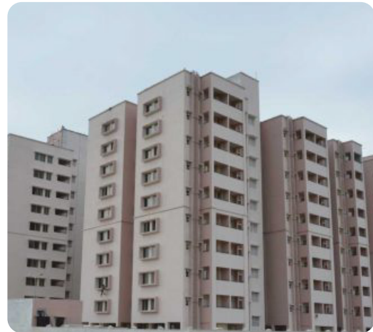
BG Shirke Project at Virar Commercial Project Firefighting Work
